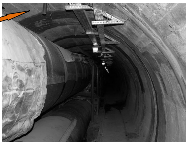
Fig. 2. General view of investigated tunnel
