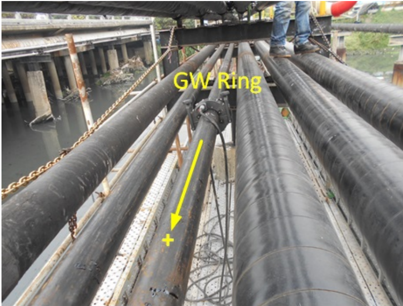
Fig. 8 Case II: 4 inch pipe CUS Inspection by GWT
