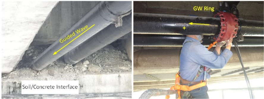
Fig.10 Case III: 6 inch pipe SIC Inspection by GWT
